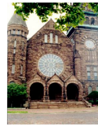
Central Congregational Church— 60 Public Square
