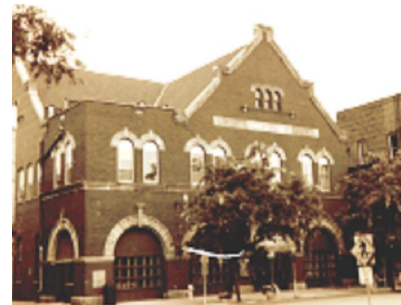
Old Central Fire Station— 150 E. Simmons St
